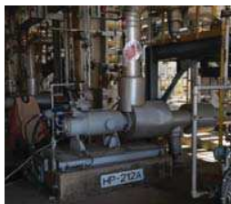
ACH leakage at flange 8" of discharge HP – 212A and found injury persons.
